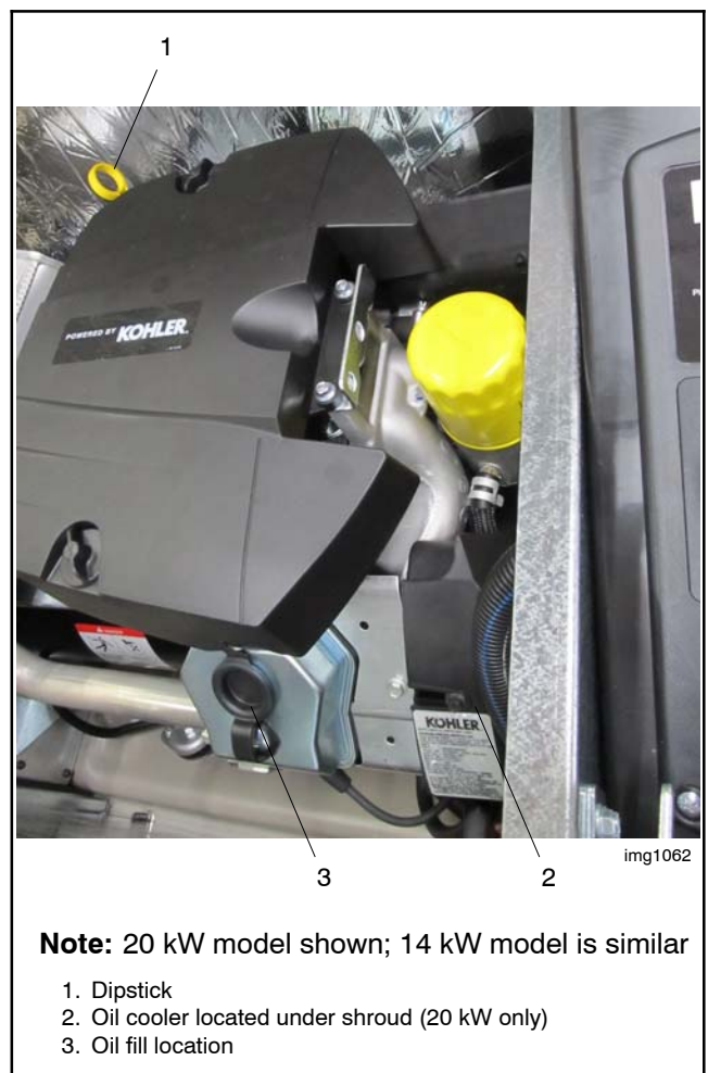
Figure 4-3 Oil Fill Components
